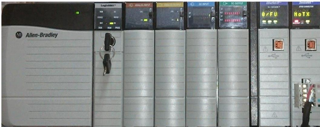
**Fig 3.** ControlLogix 5561
