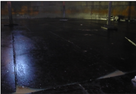
Foto 5. Paredes Tanque Fuel Oil
