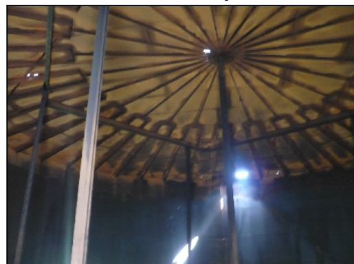
Foto 8. Paredes Tanque Fuel Oil
