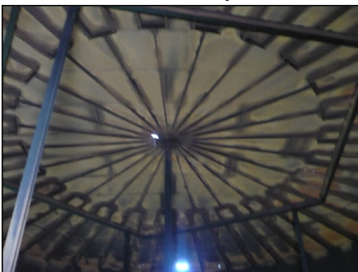
Foto 7. Paredes Tanque Fuel Oil
